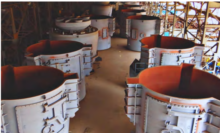
View of Heavy Fabrication Shop
